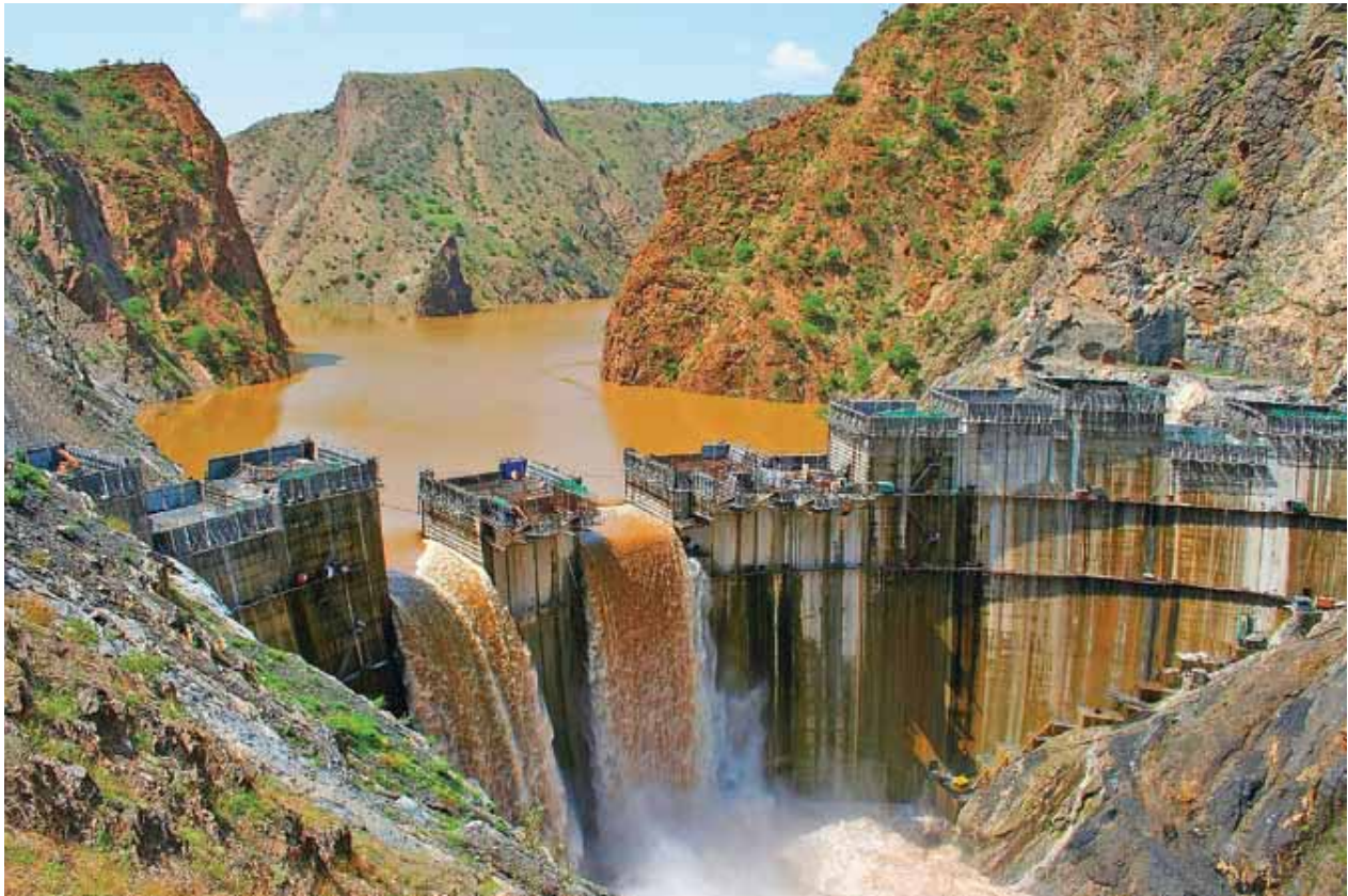
▲ The Tekezé Dam is a double-curvature arch dam in the Tigray region of northern Ethiopia on the Tekezé River, a Nile tributary that flows through one of the deepest canyons in the world. The dam consists of four turbines, together generating 300 MW. ©Paul Snook
